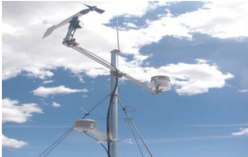
North Pump House Meteorological Station, White Mesa, Utah
